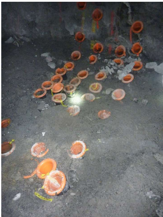
FIG 1 – Double-dip fan drilling of 100 mm blastholes in stope 0440-05050-357.
